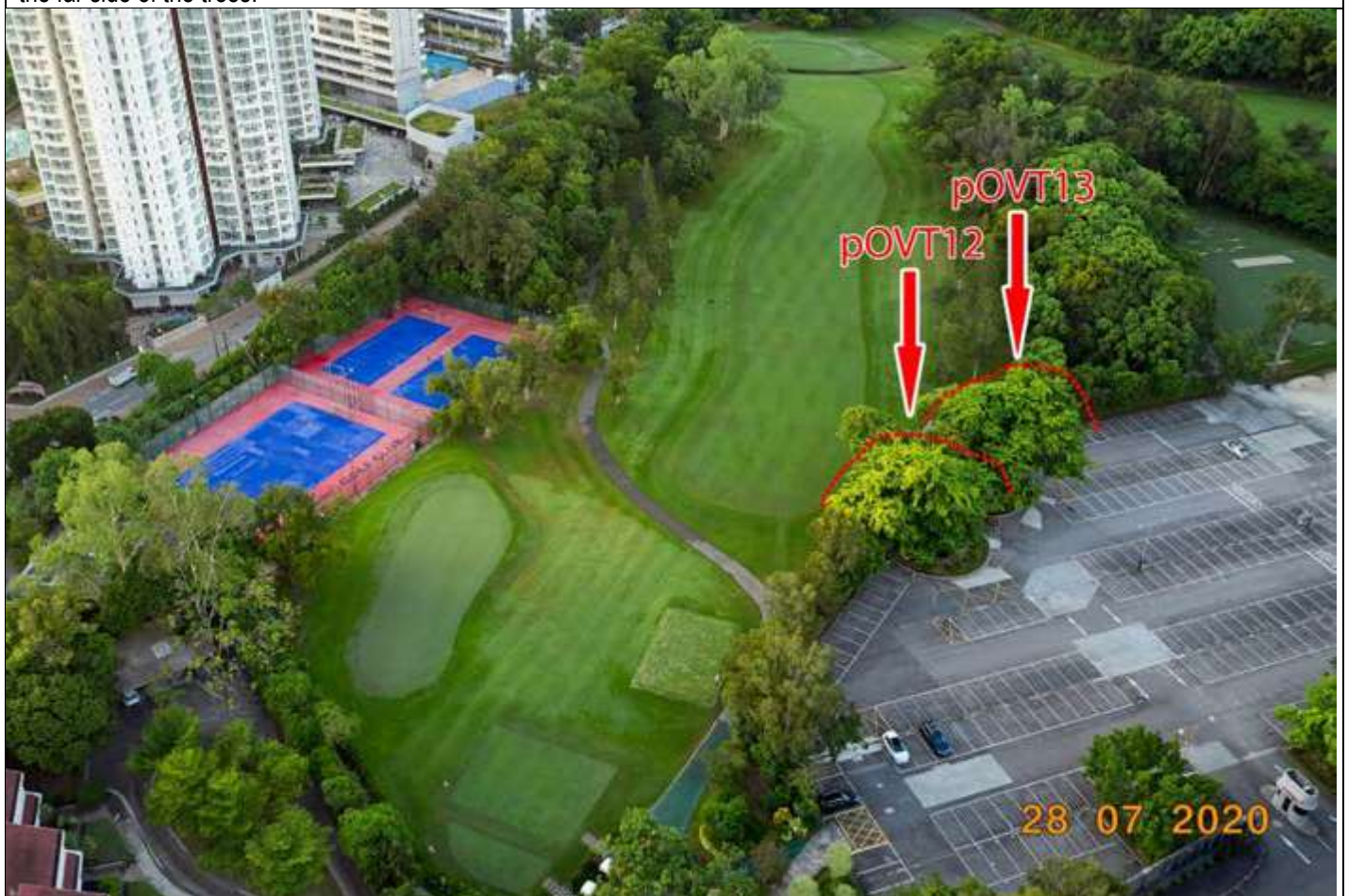
pOVT13 (View 7): The huge canopies pOVT12 and pOVT13 provide important visual separation between the first fairway of the Old Course and the HKGC car park.
