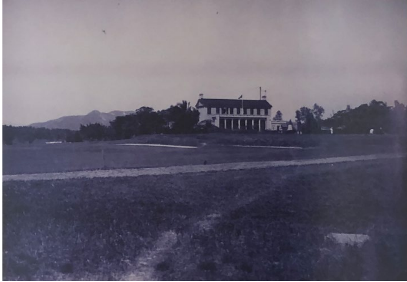
Fig. 17. Men's Club house & 18 th Green Old Coue, 1930. 65
